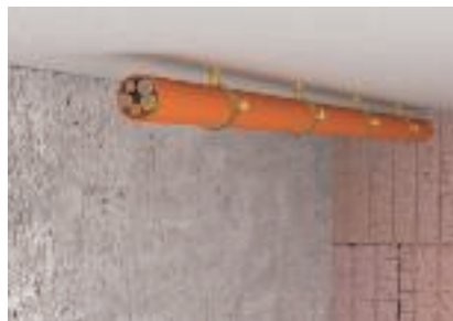
Installation under taket
